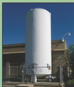
Pratliperl used to insulate Cryogenic tanks
