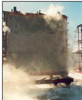
Condition of panels after application of hose stream.
