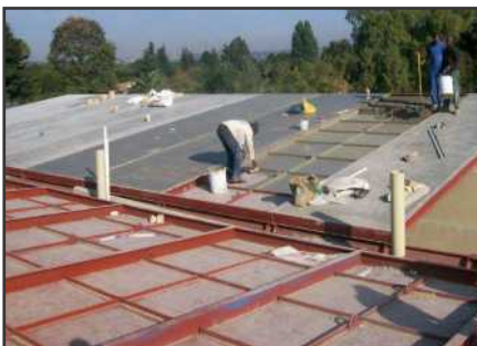
Thermally Insulating roof decks.
